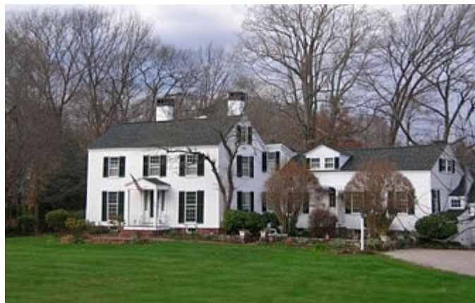
Mason House, 1303 Massachusetts Avenue
